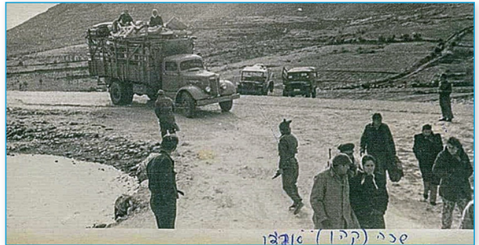
Laying Pipelines, Kibbutz Sasa 1949
